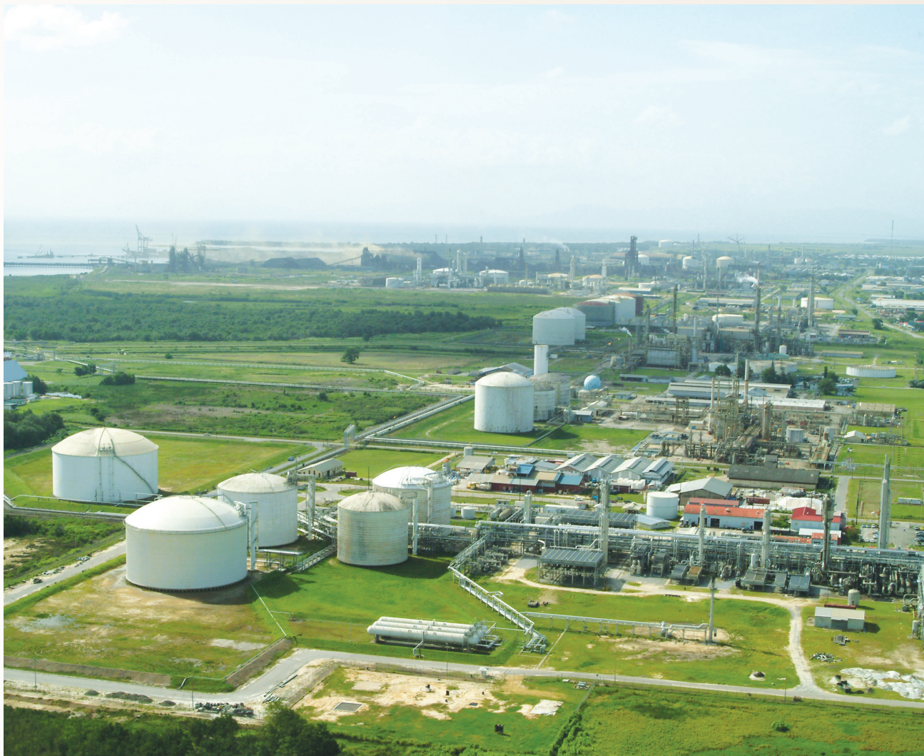
The PPGPL facility at Savonetta
